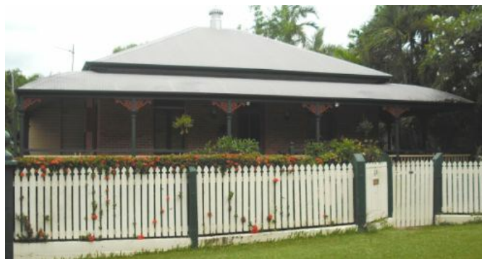
Figure SC6.2.3.9 Illustrates an example of an open front verandah, Grand Queenslander style
